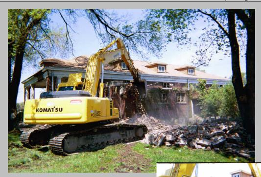
**DVG** prepared the plans and specifications for the demolition of the Wicker Park Pool & Bath House, an old WPA project constructed in 1939. DVG created the demolition construction plans, project specification, contract documents and served as the onsite construction manager during the demolition process.
